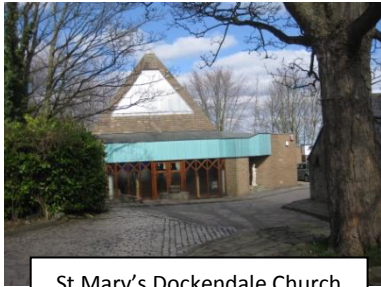
St Mary's Dockendale Church
